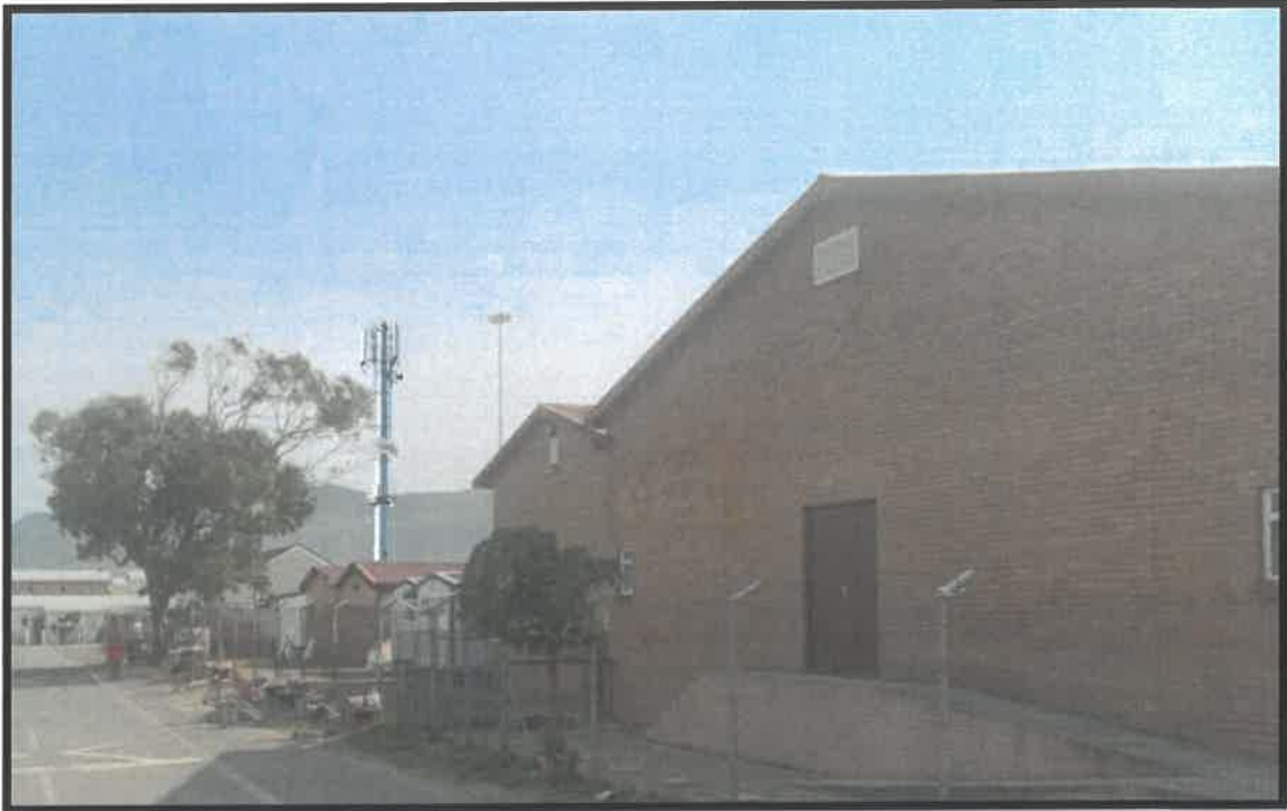
Figure 17 -- 25m Monopole mast viewed from Nama Street
