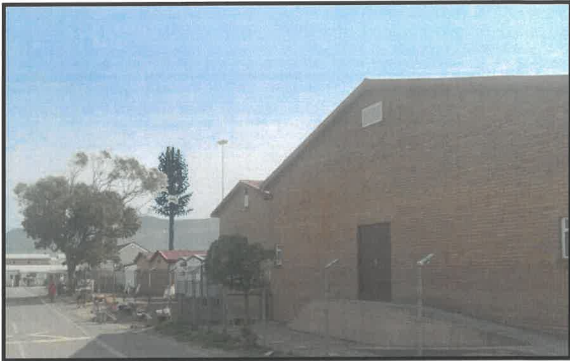
Figure 19 - 25m Tree mast viewed from Nama Street
