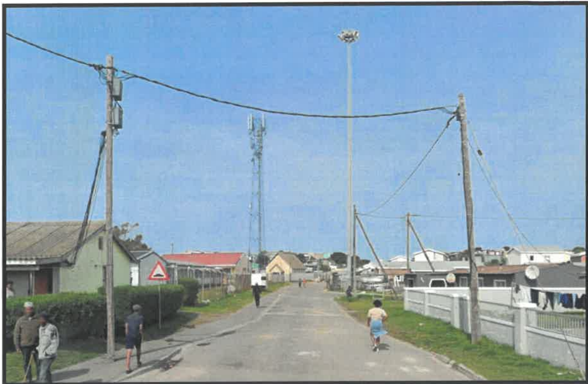
Figure 14 – 25m Lattice mast viewed from Hlobo Street
