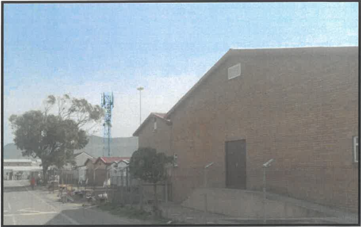
Figure 15 – 25m Lattice mast viewed from Nama Street
