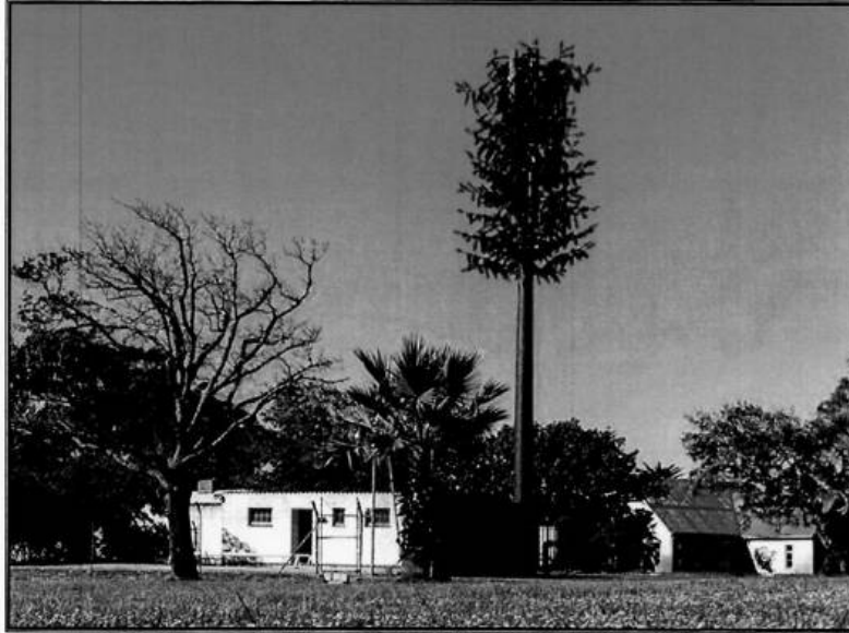
Fig. 12 – Example of tree type land-based transmission apparatus built by our client
