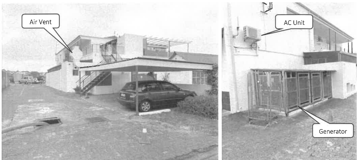
Figure 10: Existing Infrastructure creating noise
