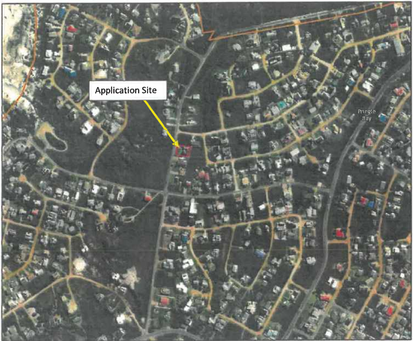
Figure 2: Aerial Photograph of application site and surrounding area (Cape Farm Mapper, April 2022)
