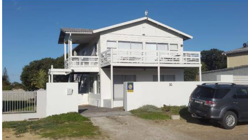
PHOTO OF CURRENT RENOVATED PORCH DIRECTLY BENEATH OPEN WOODEN DECK
