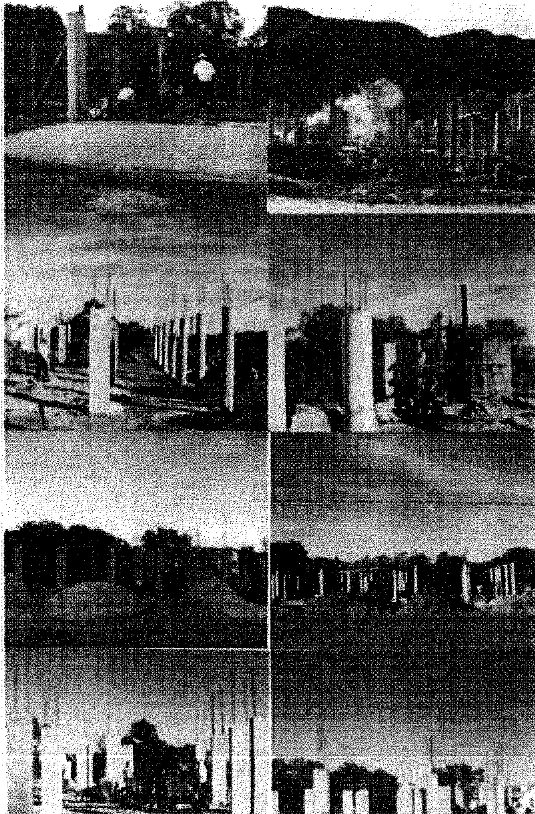
PIC 14 the construction of Oude Schuur in 1985
