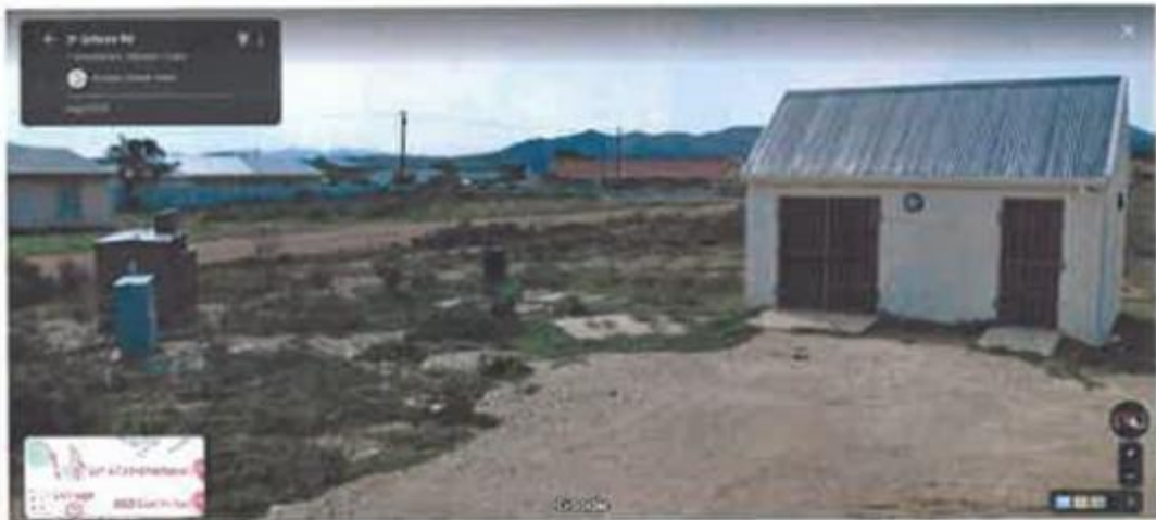
STREET VIEW OF PUMP STATION
