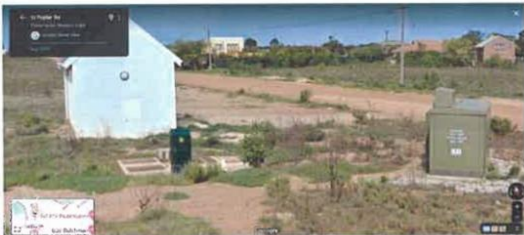
STREET VIEW OF ELEC SUBSTATION
