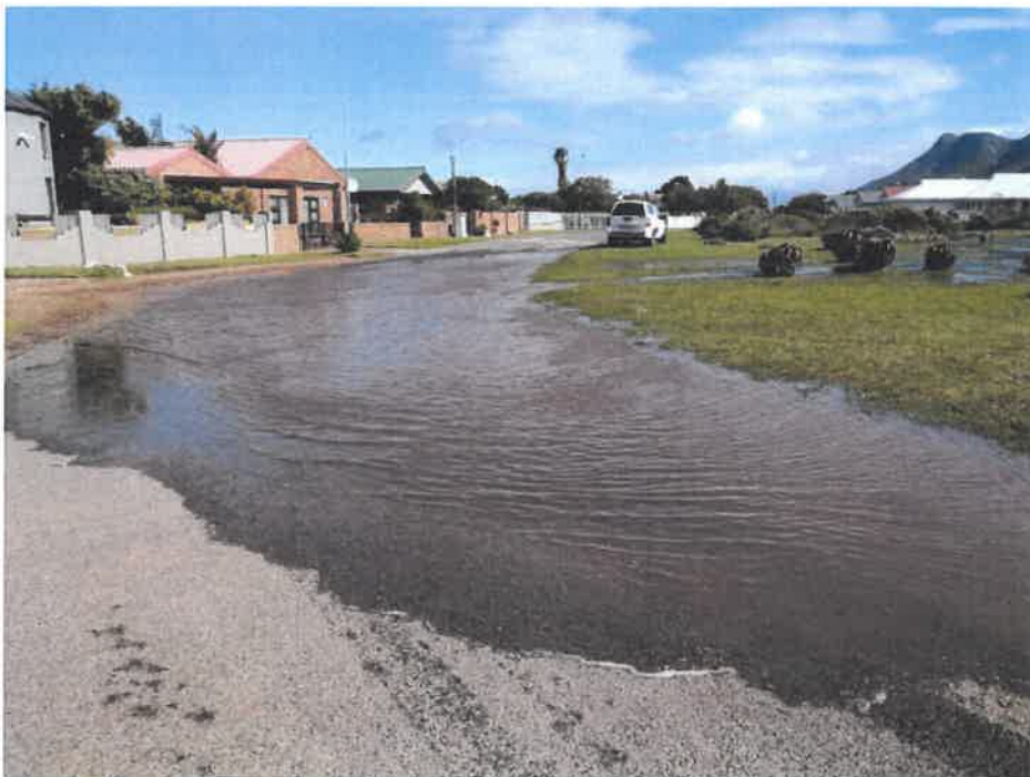
Figure 3 A typical situation where rain water drainage is ineffective in Sandbaai
