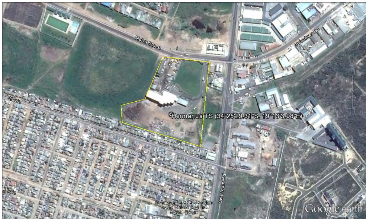
Figure 3-13: Hermanus Solid Waste Transfer Station & Material Recovery Facility (MRF)
