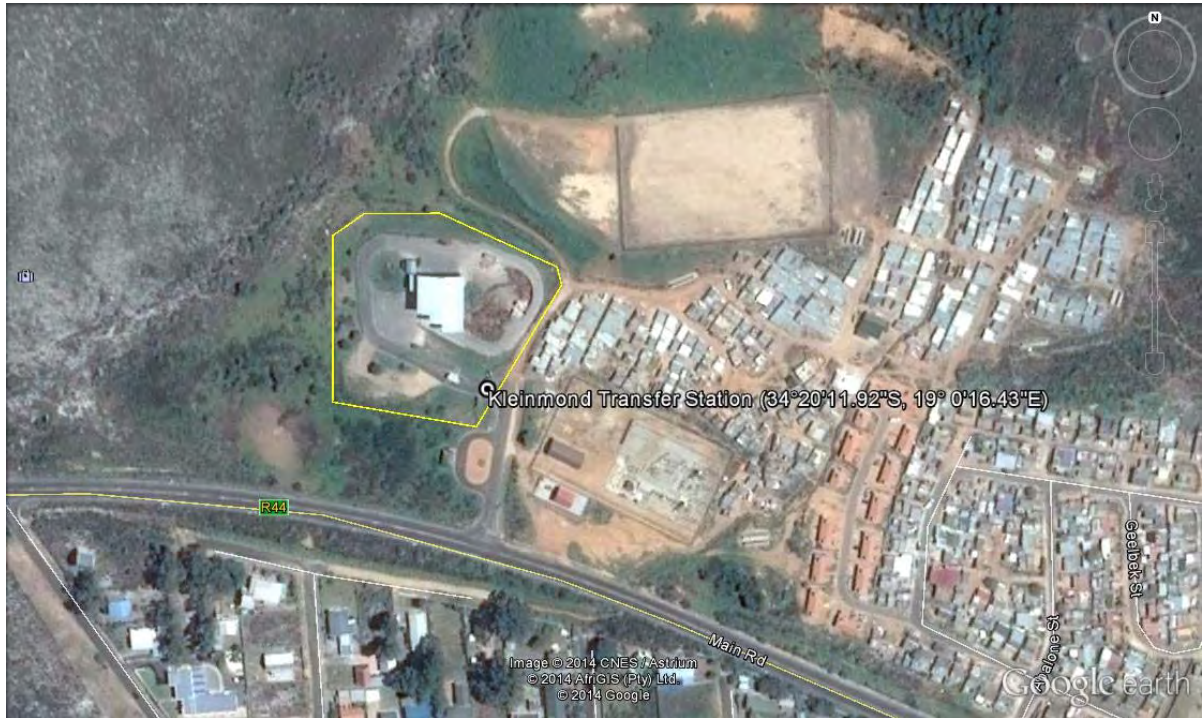
Figure 3-14: Kleinmond Solid Waste Transfer Station
