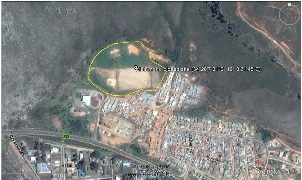
Figure 3-12: Kleinmond Rehabilitated Disposal Site
