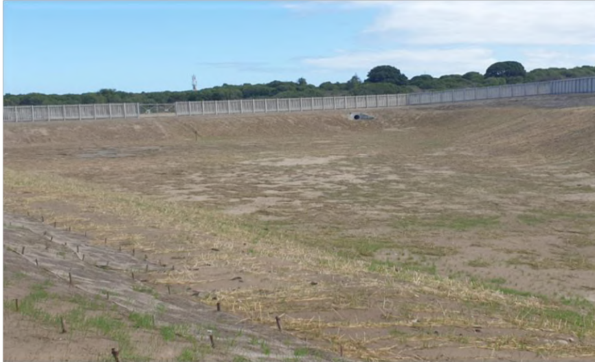
Masakhane Stormwater Pond
