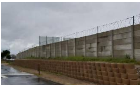
Retaining wall in 9 th Avenue Kleinmond to create space for construction of sidewalk
