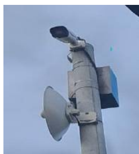
CAMERAS BEING INSTALLED ACROSS THE OVERSTRAND JURISDICTION
