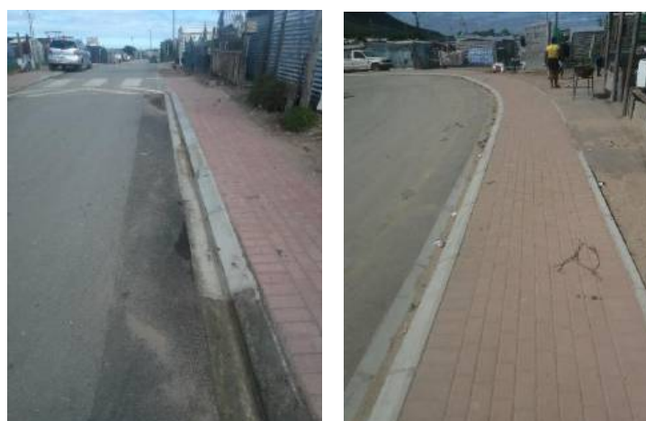
Construction of Sidewalks in Masakhane, Gansbaai (Phase 2)
