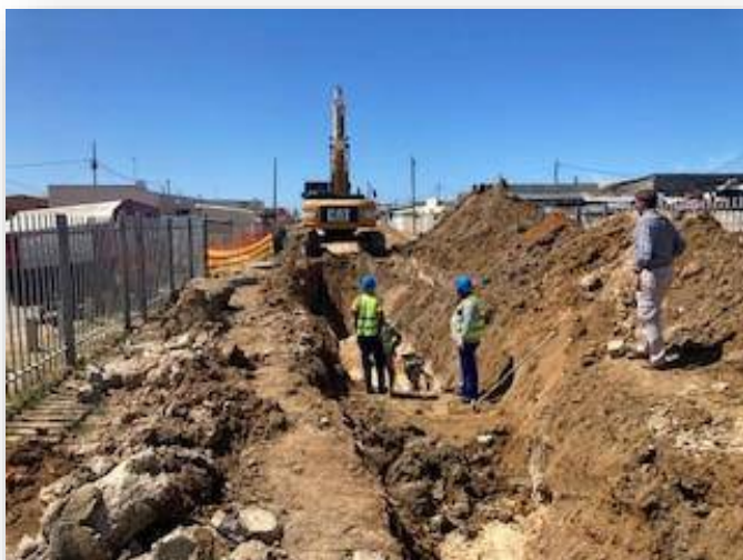
Extension of the sewer network in the Mountain avenues of Kleinmond
