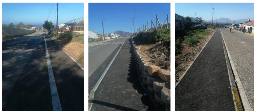
Construction of Sidewalks in Proteadorp, Kleinmond (Phase 2)
