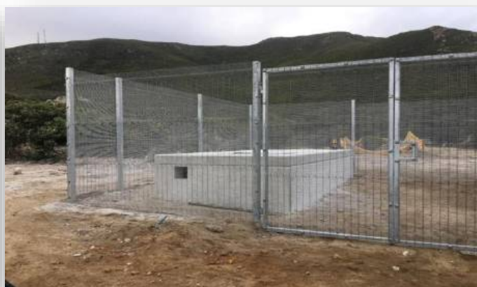
New production borehole at the Gateway well field, Hermanus
