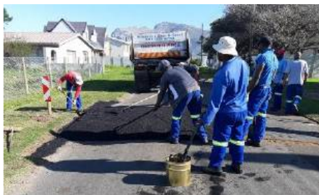
Installation of speed humps in Kleinmond
