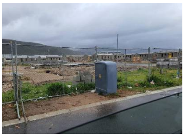
Electrification of new houses are in progress at Swartdam C1.
