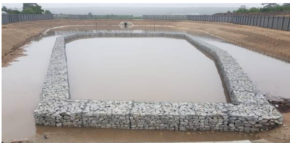
Stanford Housing project Stormwater Pond
