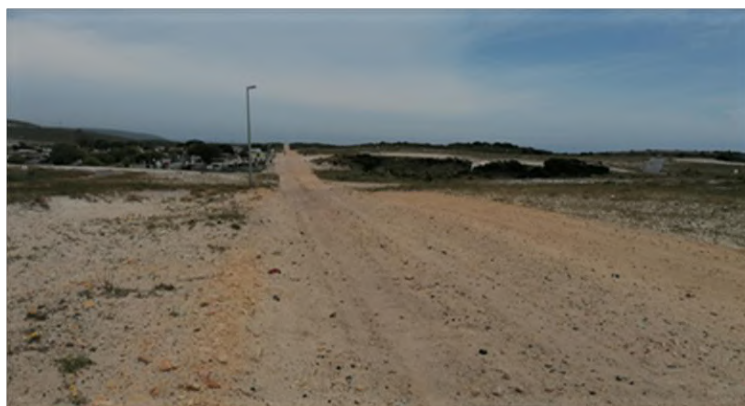
Road to be upgraded
