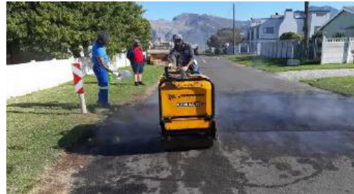
Installation of speed humps in Kleinmond
