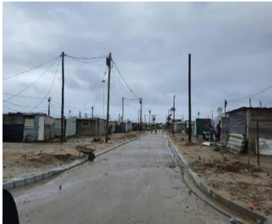
Re-electrification of households in Zwelihle Transit Camp
