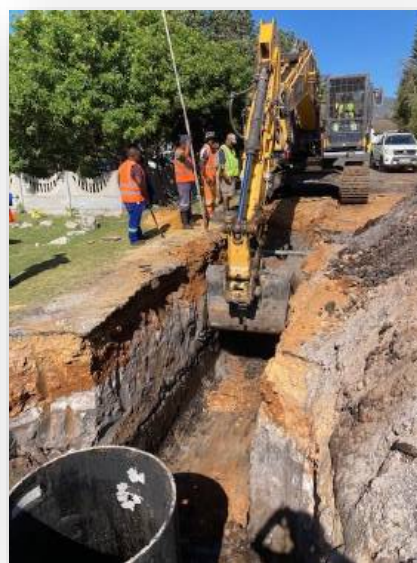
Upgrade of the main sewer in the Sipumelelo Corridor, Zwelihle, Hermanus
