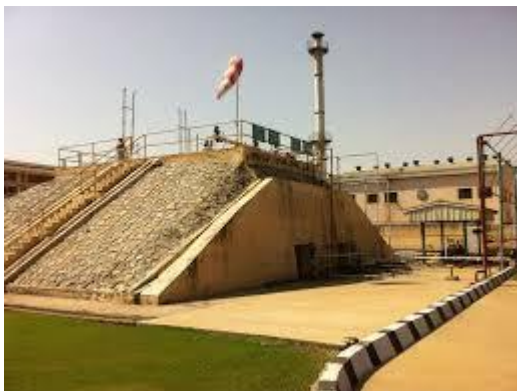
Example of a mounded tank facility
