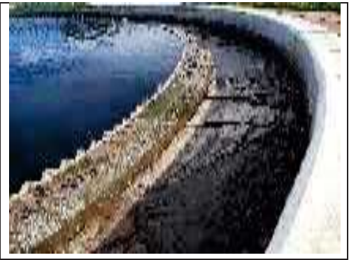
Flow distribution uneven and deliver high flows to 1 of 4 clarifiers. Work done during TSA to rectify this design defect.
