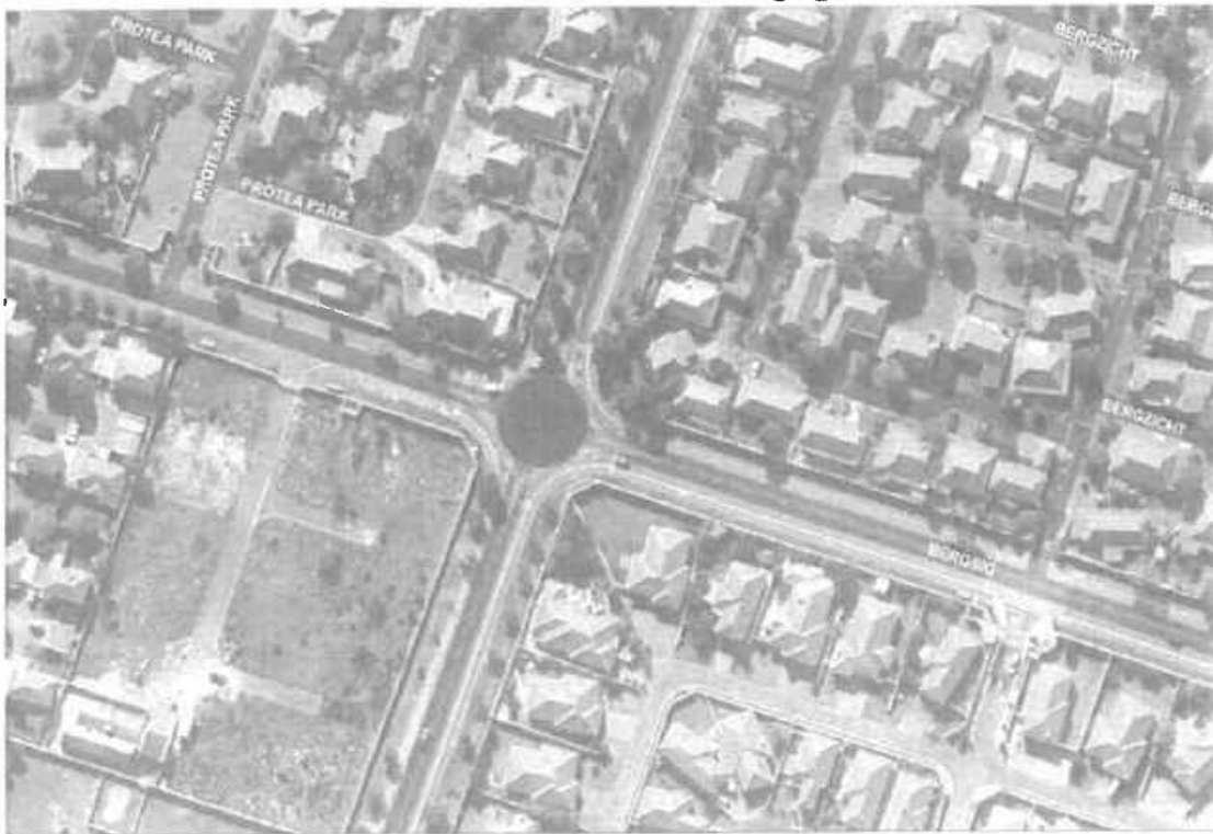
Site 9: PTZ Camera and LPR at Sandbaai Main Road / Bergsig Traffic Circle
