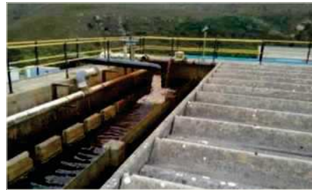
KMnO 4 treated water entering settling tank - Chemical Oxidation Treatment- Preekstoel WTW
