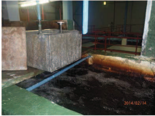
Gravity flow dosing system of flocculent
