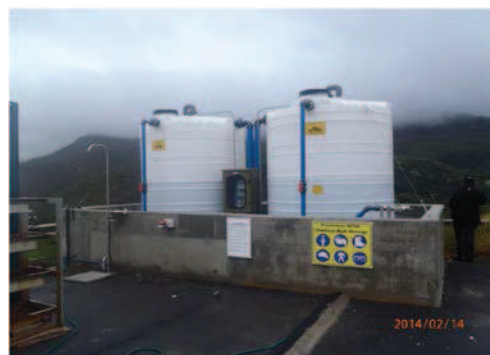
Bunded area for chemical storage tanks
