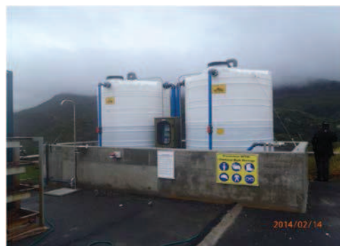
Bunded area for chemical storage tanks
