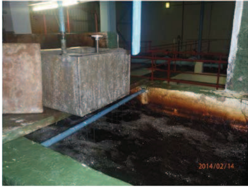
Gravity flow dosing system of flocculent
