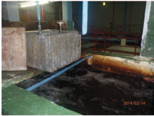
Gravity flow dosing system of flocculent
