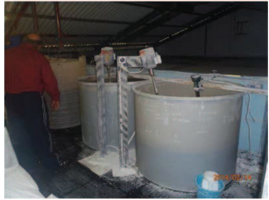
Chemical tanks not banded
