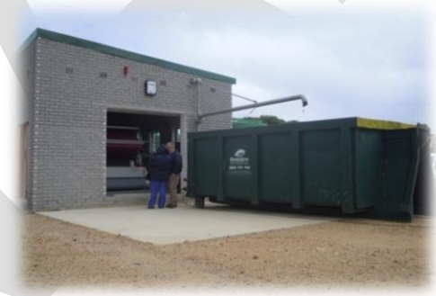
Gansbaai Waste Water Treatment Works (WWTW) Sludge handling facility
