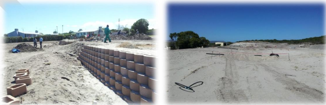
Preparation of site and installation of services at Eluxolweni, Pearly Beach
