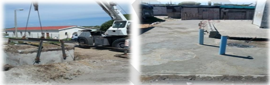
Installation of basic services in Masakhane
