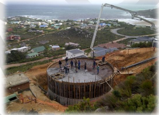
Construction of Rooiels Reservoir
