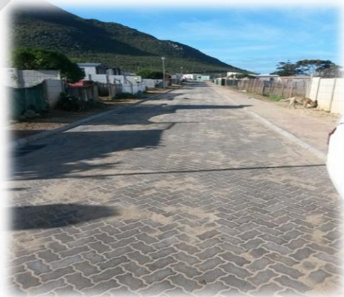
Road construction in Hawston
