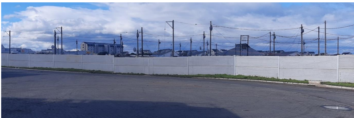
The new section of the upgraded perimeter wall at the Hermanus Transfer Station.
