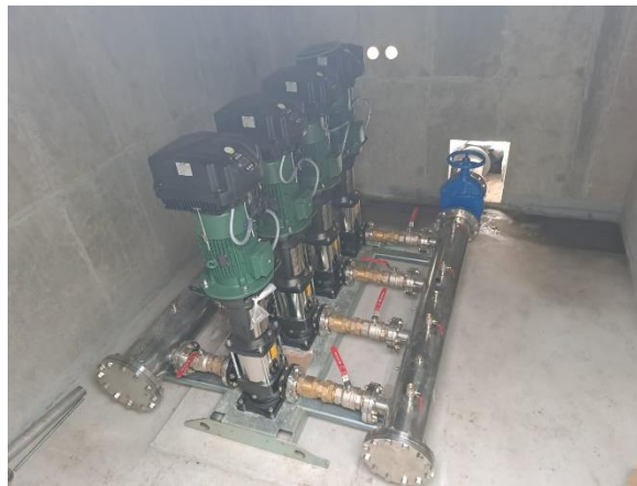
Masakhane Upgrade Waterlines & New Booster Pumpstation
