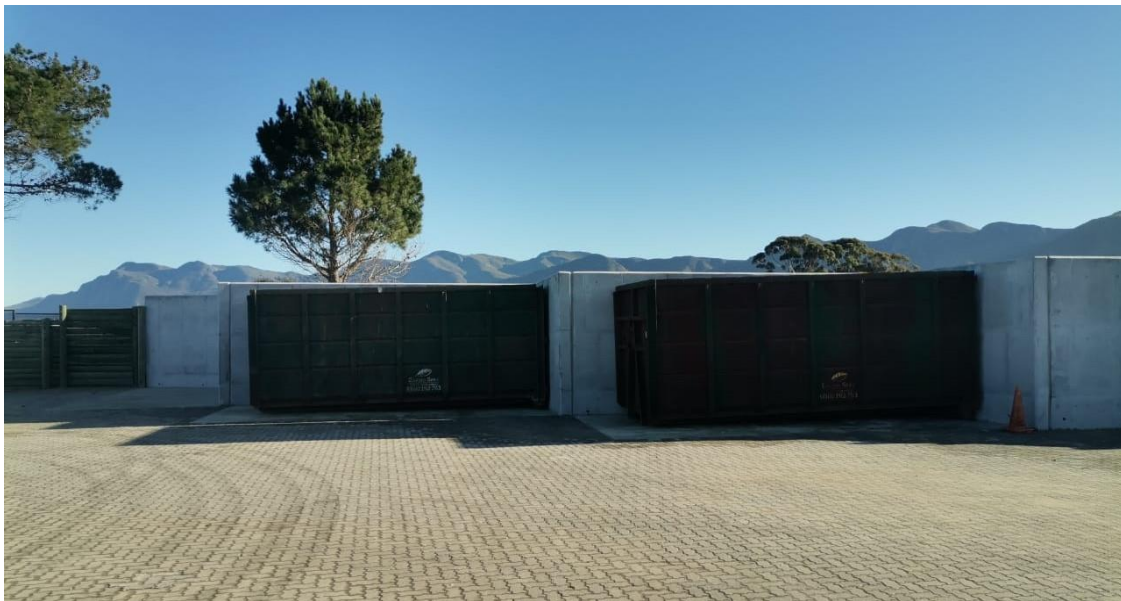
New concrete retaining walls constructed at the Stanford Drop-off site.
