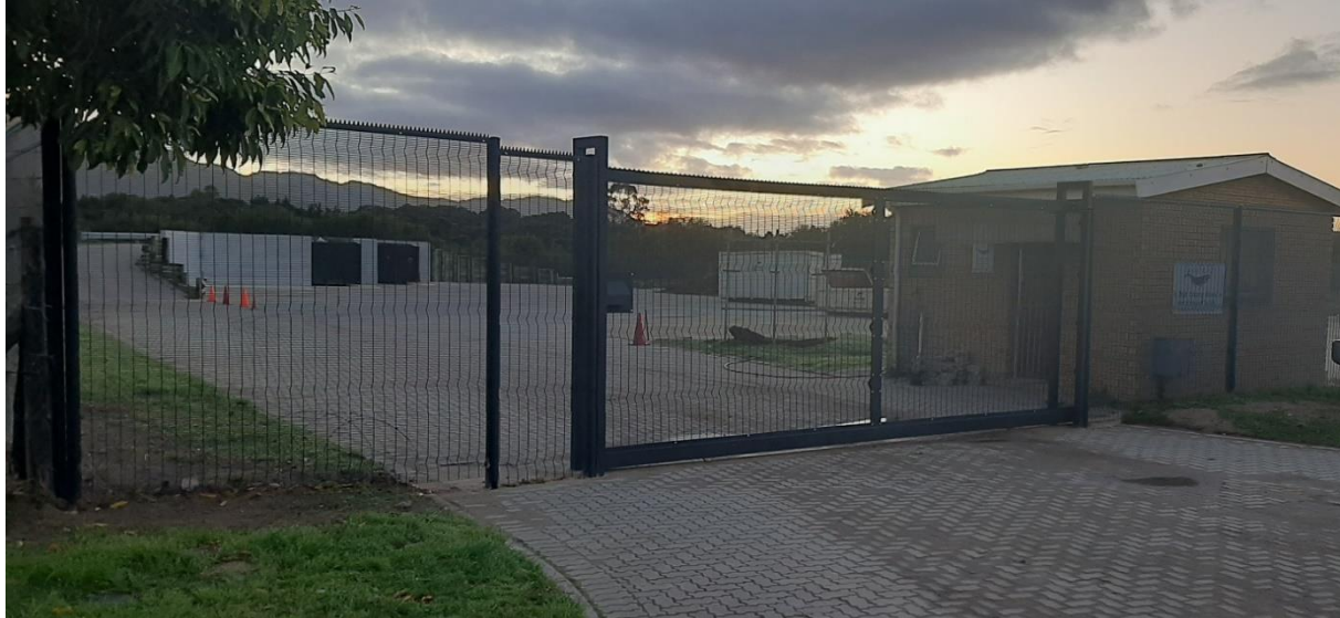
The new access gate and fence at the Stanford drop-off. Also visible is the new concrete retaining wall.
