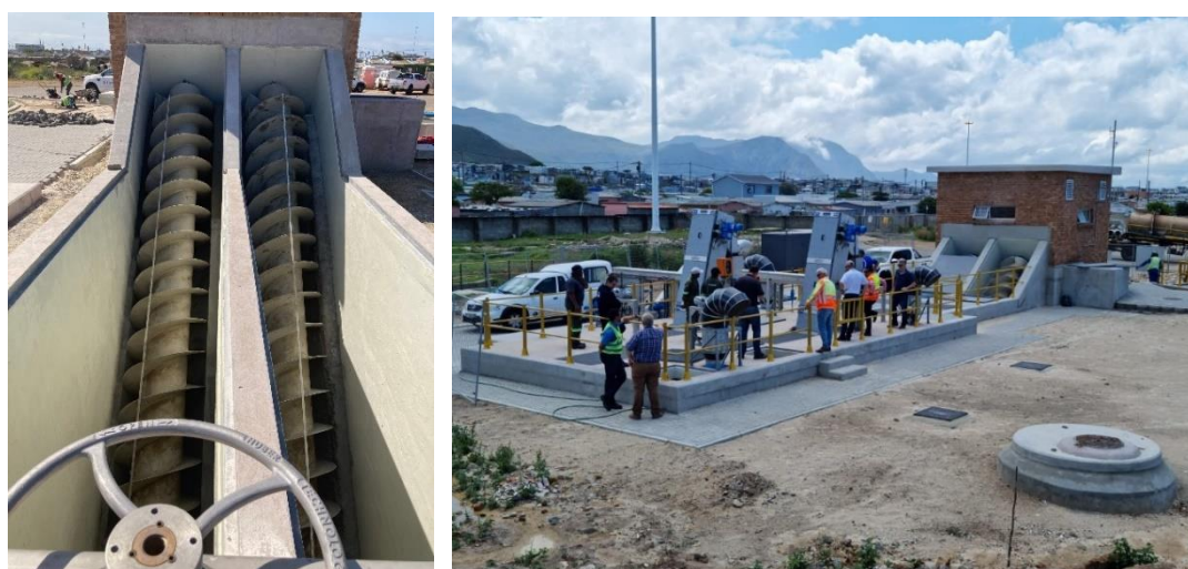
Construction of the new Archimedes Screw inlet Pump Station at the Hermanus Wastewater Treatment Plant was completed.
