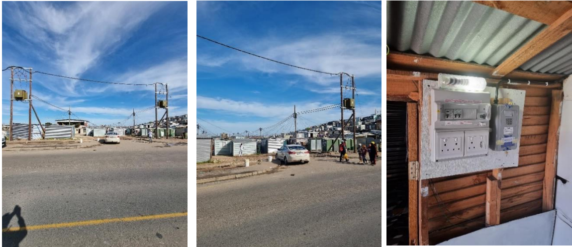
Marikana Electrification project (Phase 1) 650 informal households
