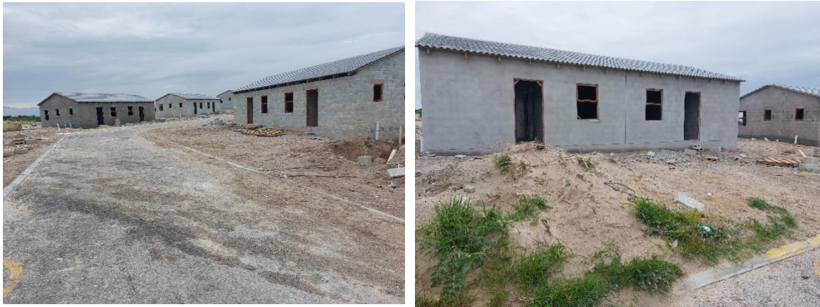
Blompark Top Structures, Gansbaai - Phase 3 – 150 Houses
