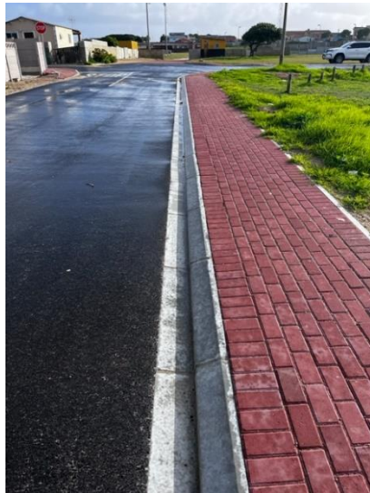
Rehabilitate Roads Blompark
