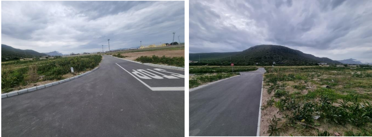
Mount Pleasant & Westdene IRDP infill sites – PHASES 1 & 2 – 215 SITES- Installation of civil infrastructure
