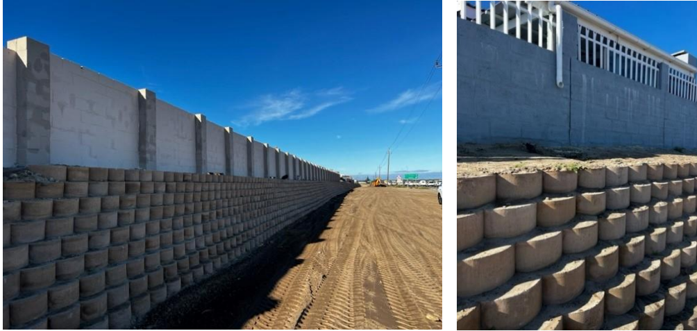
Hawston Boundary Wall
