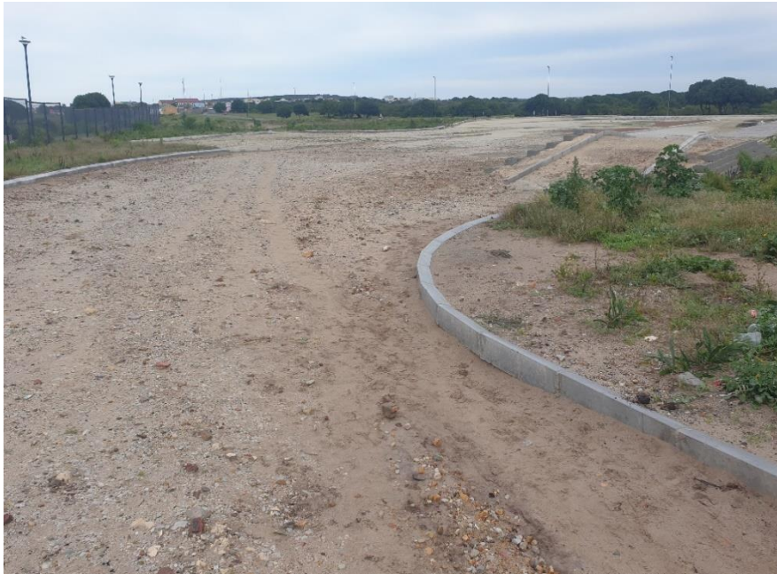
Figure 18: REPAIR DAMAGED SURFACE AND LAYERWORKS
