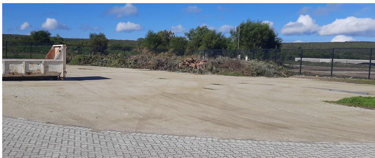
Upgraded garden waste offloading area and new fence for the Stanford Drop-off
