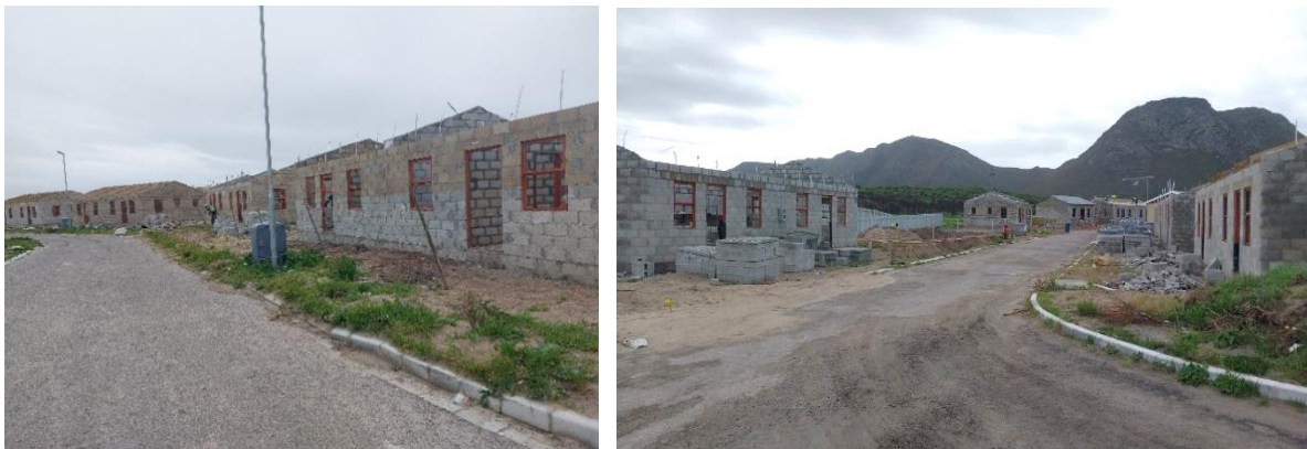
Masakhane Top Structures, Gansbaai - Phase 2 – 145 Houses
