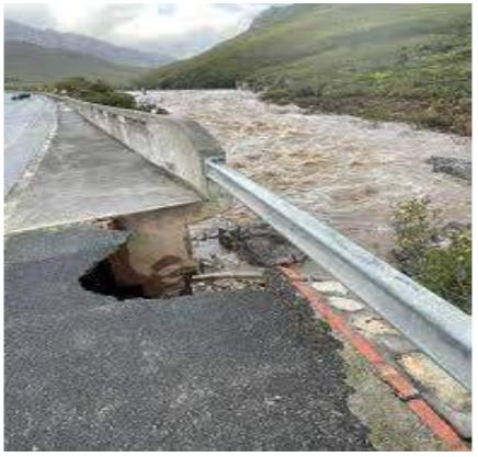
Figure 20: Flooding damage at Kleinmond bridge
