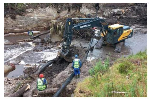
Figure 21: Pipeline repairs to damaged infrastructure
